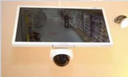
Live CCTV Installation
